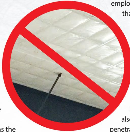
Unfortunately, many existing arenas and even new arenas employ permeable fiberglass batt-style insulation that is contained by an impermeable membrane below. This membrane impedes vapor from dissipating so the humidity above it is too high. Because the cold ice surface chills down the structure above, condensation results above this membrane and ultimately drips out onto the ice.
