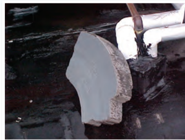
Catastrophic Media Failure
