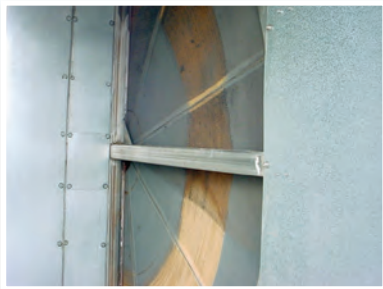
Mechanical Failure Rotor Appearance
