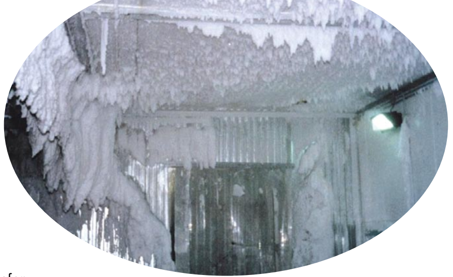
Fogging from the moisture infiltration through the pallet door.
