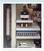
Combination circuit breaker/overload starters for fan motors eliminates the need for spare power fuses and saves downtime. If an upset occurs, a simple reset will bring the unit back online.
